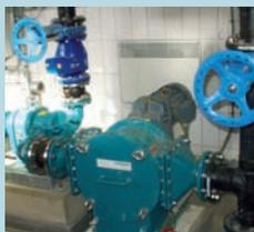
In a Wastewater Treatment Plant the thickened sludge is pumped to a centrifuge. The sludge contains large quantities of solids, fibers and rags. To avoid blockages to the centrifuge and to protect the pumps, a Multichopper P300-I was installed in the suction line of the Börger pumps. Fibers, solids and rags in the sludge are chopped down and within the same operation the sludge is homogenized.
