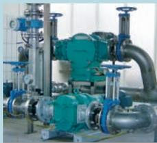
In a municipal sewage treatment plant the wastewater is filtered by use of membrane technology. The membranes separate the sewage into permeate (filtered water) and sludge. The sludge is temporarily stored in large tanks. A sludge loading station equipped with a Börger Multichopper and a Rotary Lobe Pump will fill up tankers in minimal time for transfer to a dewatering station. The Multichopper protects the pump and the downstream dewatering equipment by reducing the solids size.
