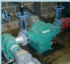
Food and garden waste are delivered to a biogas plant and are mixed with liquid. The Börger Multichopper and a Börger Multicrusher are installed to chop the solids and homogenize the product. Börger pumps transport the mass to an anaerobic digester. With the combination of the both Börger chopping machines the required solids size necessary for biogas plants are achieved.
