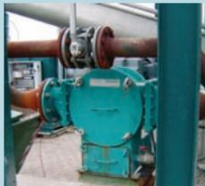
Spent vegetable oils and deep-frying fats are reconditioned in a Biodiesel Plant. The Multichopper reduces large solids to enable them to be separated easily in the downstream processes. The cleaned oils and fats are pumped to large Diesel-Engines driving generators for energy production. The Multichopper is handling a range of 400 usgpm with a maximum temperature of 140 °F.
